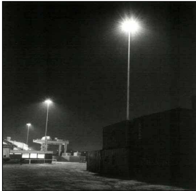
Figure 15 Floodlighting, by predominantly downward lighting, of an area where obstruction can occur
