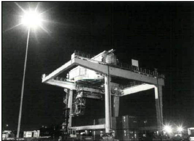
Figure 17 Floodlighting by projectors of an area free from obstructions
